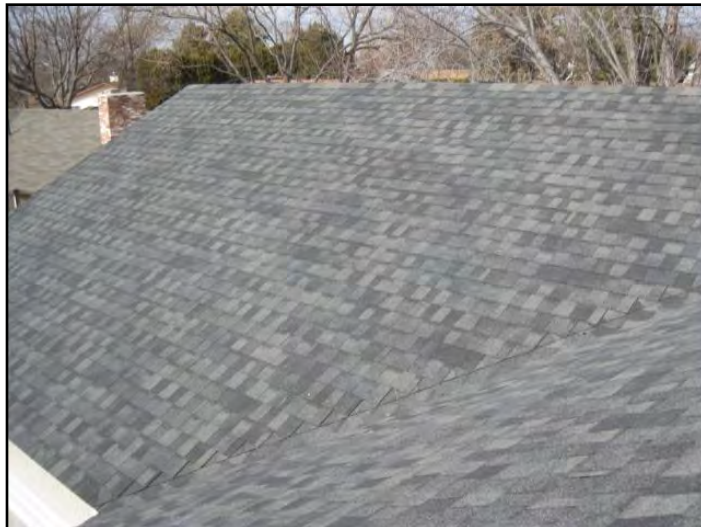
2. The roof is in average condition for a home...
