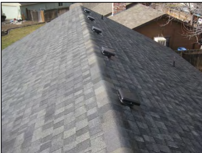
3. The roof is in average condition for a home...
