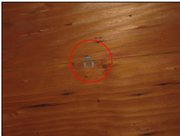
4. Hurricane clips observed
