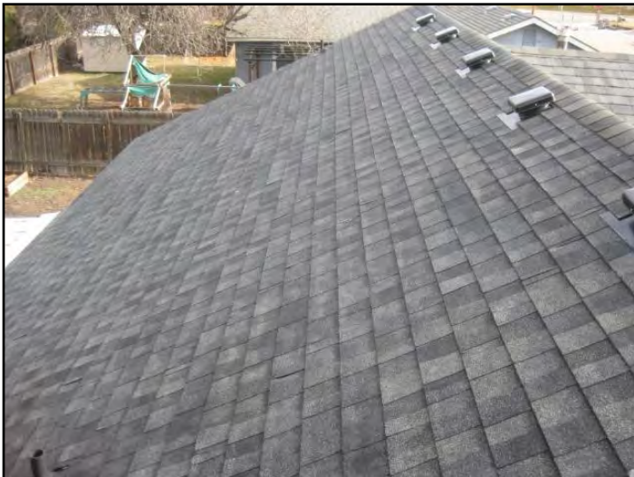
1. The roof is in average condition for a home...
