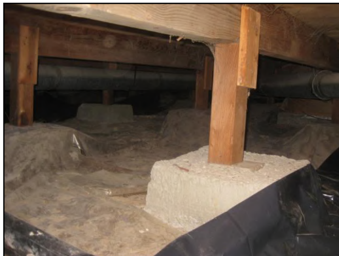
16. Wood columns on concrete piers
